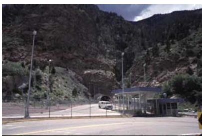
NORAD Facility entrance
